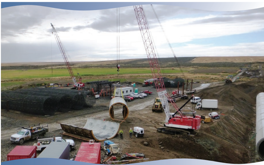
Crane lifting inside form, rebar fabrication yard in the background.
