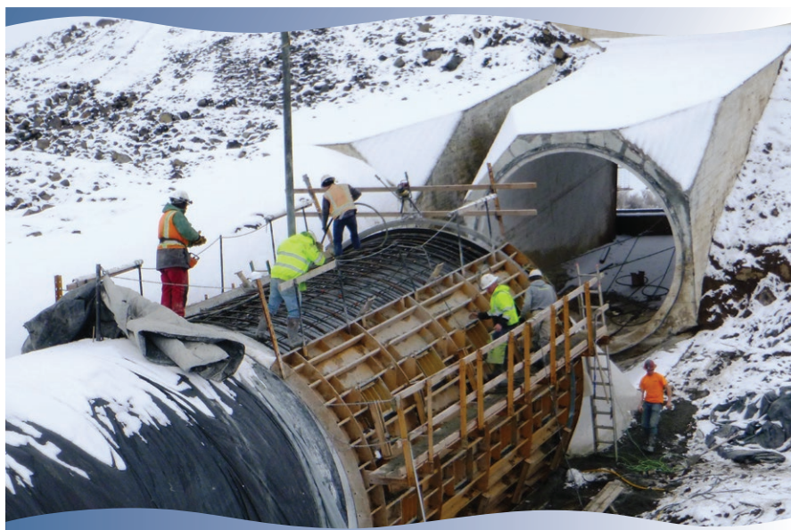
Concrete placement near existing inlet structure of Lind Coulee Siphon Number 2.
