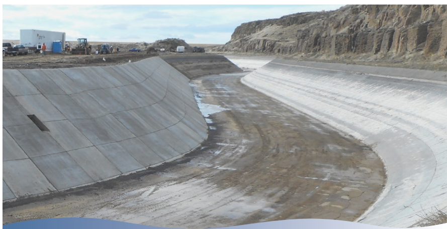
View of replaced panel sections on Main Canal in QCBID.
