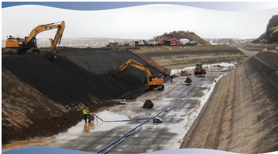
Demolition of cracked Main Canal concrete panels near F Road Northeast.
