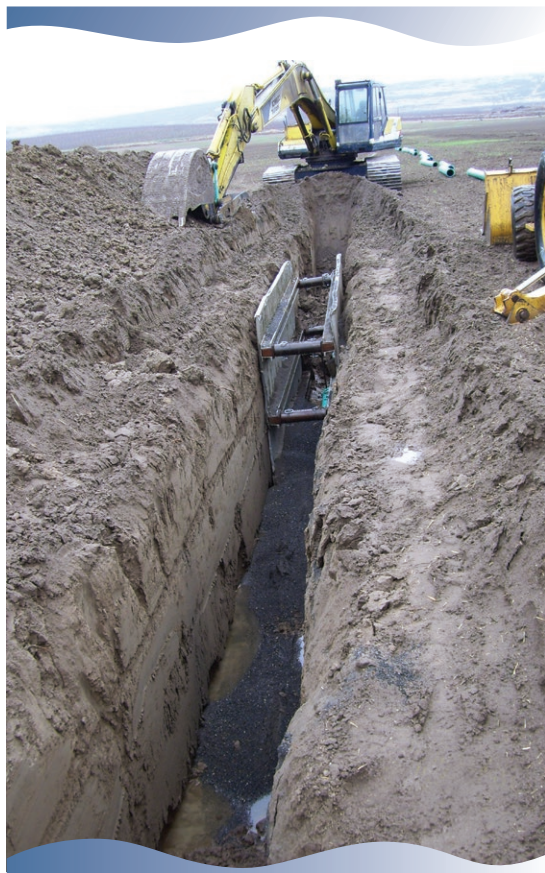
QCBID Subsurface Drainage project.
