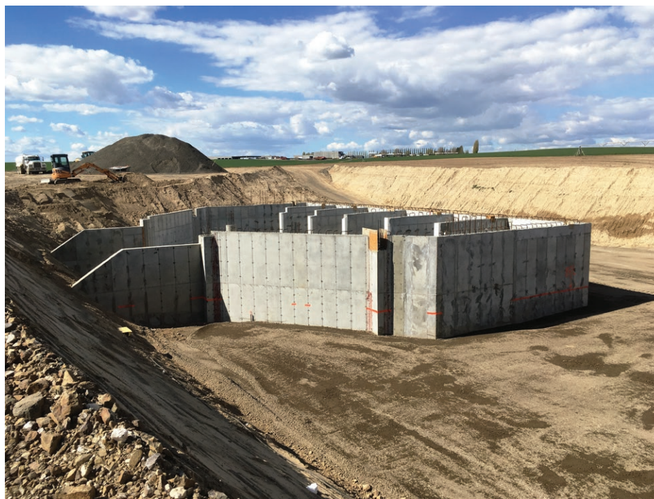
East Columbia Basin Irrigation District's EL 47.5 pump station construction progress.
