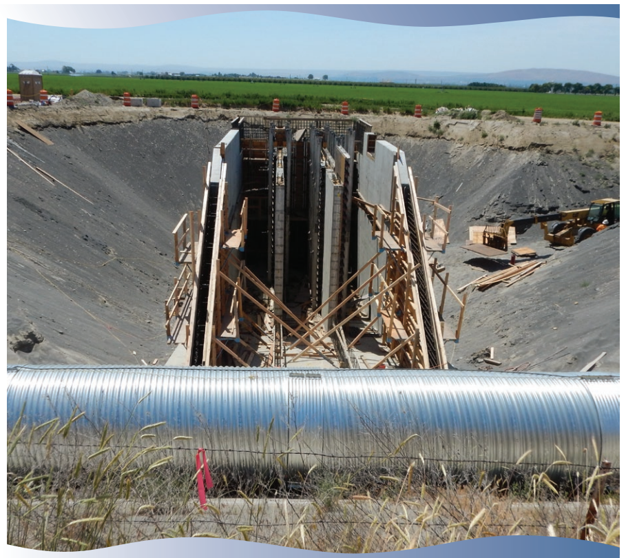
Construction at the PPL1.6 Pumping Plant.
