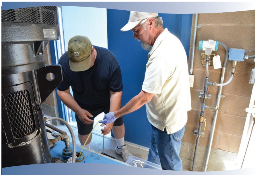
Charlie Brown (Left) with Evergreen Rural Water of Washington assists a staff person from the City of George with well measurement.
