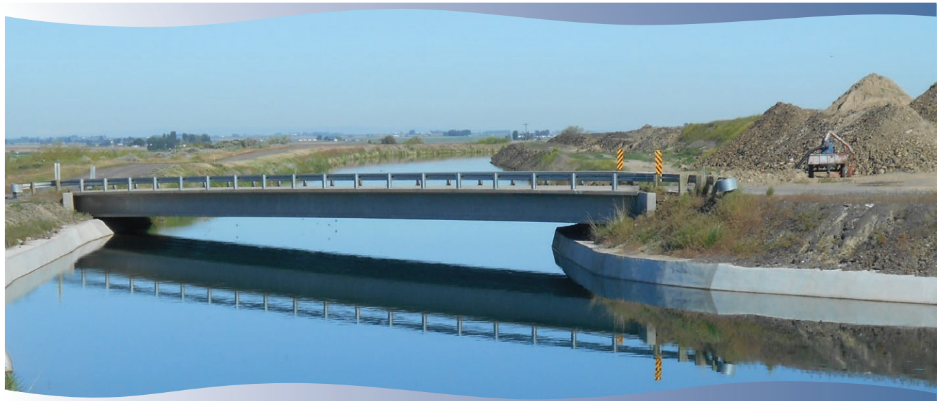
At Calloway Bridge in Adams County; due to the design and relative newness of the bridge, ECBID was able to make key updates rather than replace the bridge entirely.
