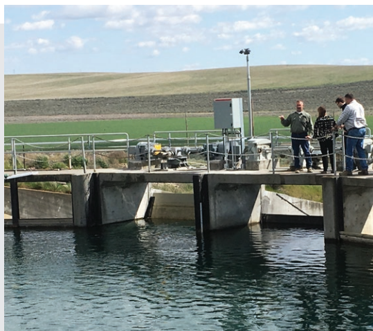
ECBID and PFM staff at the Lind Coulee Wasteway.
