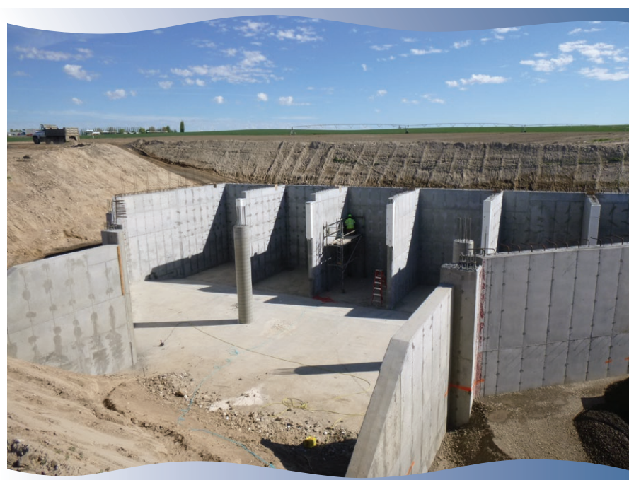
EL 47.5 Pump station site construction progress.
