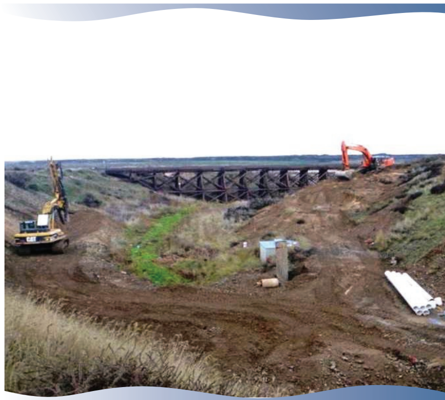
Warden Siphon Site Preparation in East Columbia Basin Irrigation District November 15, 2016.
