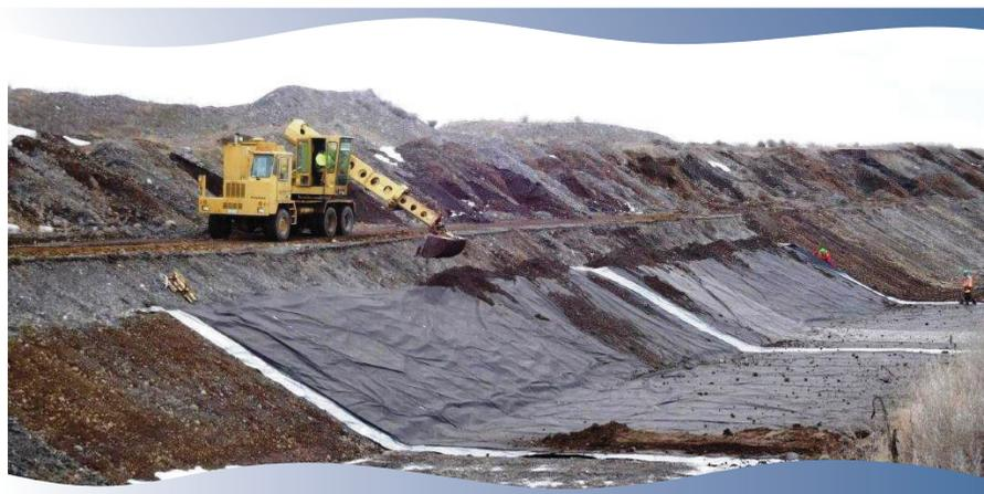
*QCBID crews buries a geomembrane liner on W20 canal in the Winchester section.*
