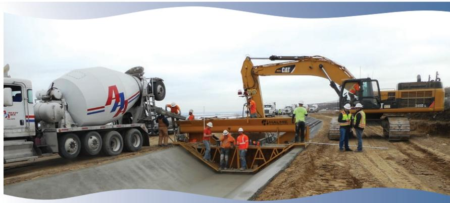
*QCBID hired contractor, Halme, places a concrete liner at W61 canal in the Royal section.*
