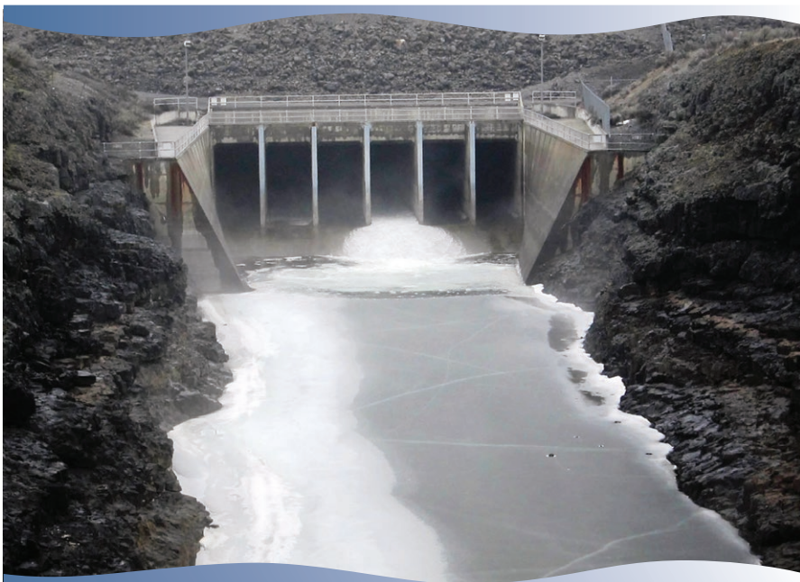
Water begins to flow from the Bank Lake headworks.
