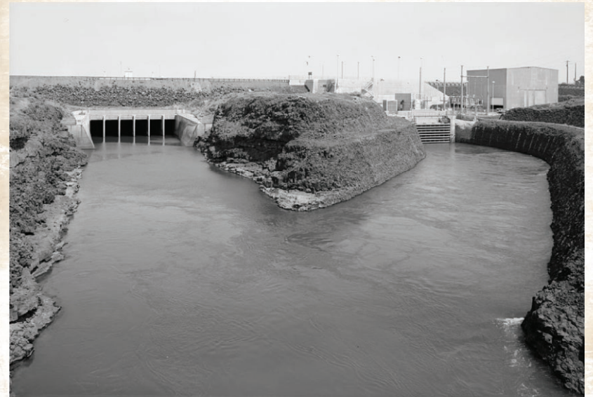
Banks Lake Dry Falls Dam & Main Canal Headworks.
