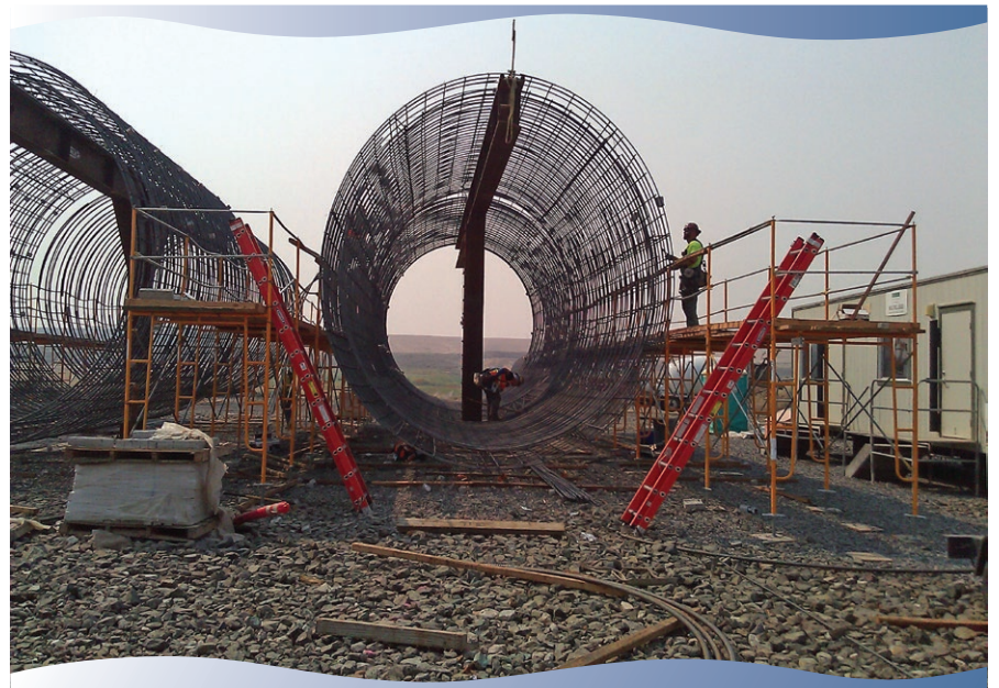
Preparation of Rebar Cage at Lind Coulee Siphon Construction Site.
