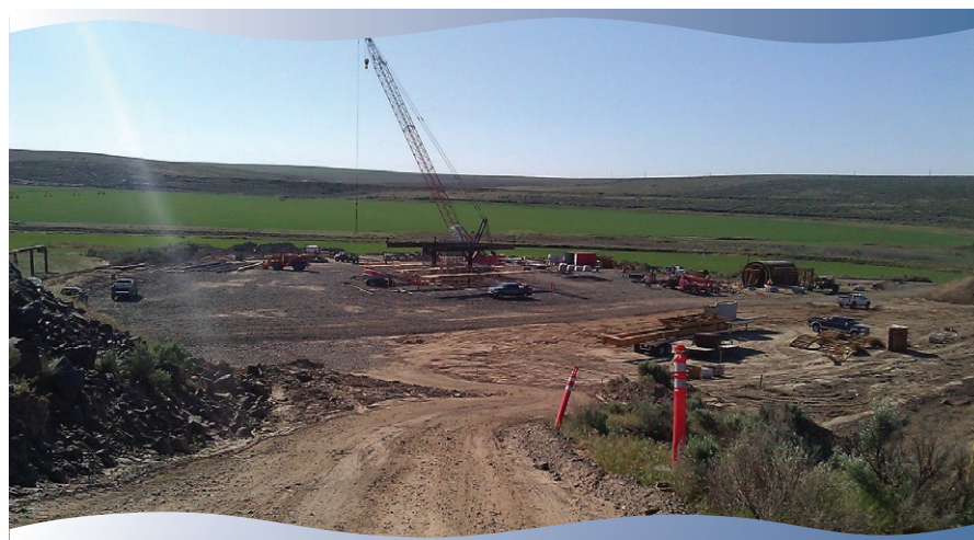
Staging area for test section construction and rebar cage formation.
