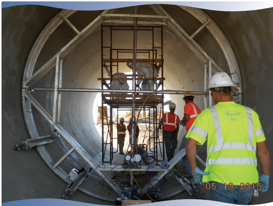
Pressure testing rubber seal in siphon test sections.
