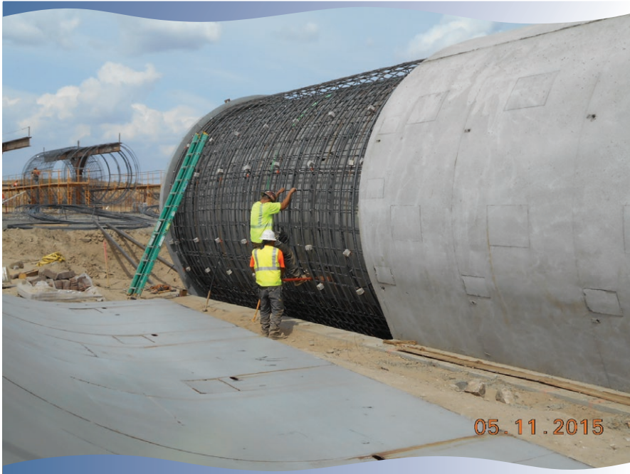
Siphon: Rebar cage adjustments before outer form is set.
