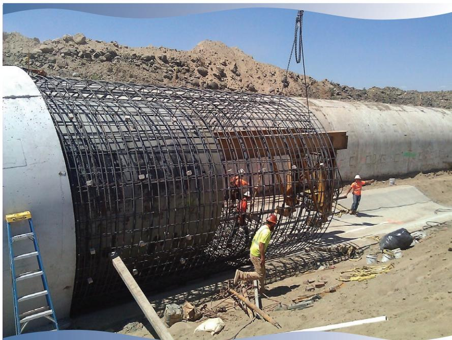
*Placement of rebar cage at Lind Coulee Siphon 2, a portion of interior form is already installed.*
