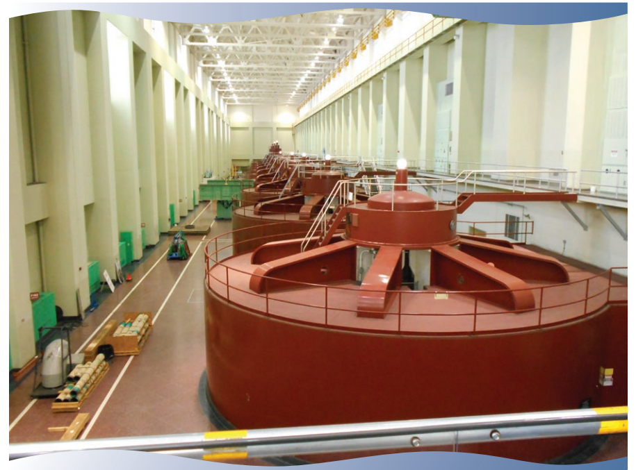
Grand Coulee Dam Left Power House.
