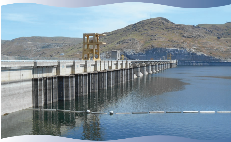
View of Grand Coulee Dam Pump Generating Plant.
