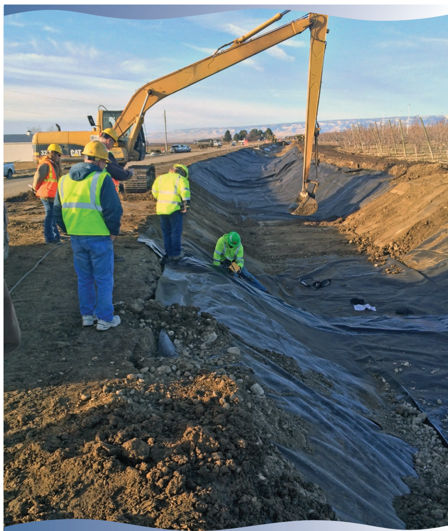
Geomembrane Installation in QCBID.
