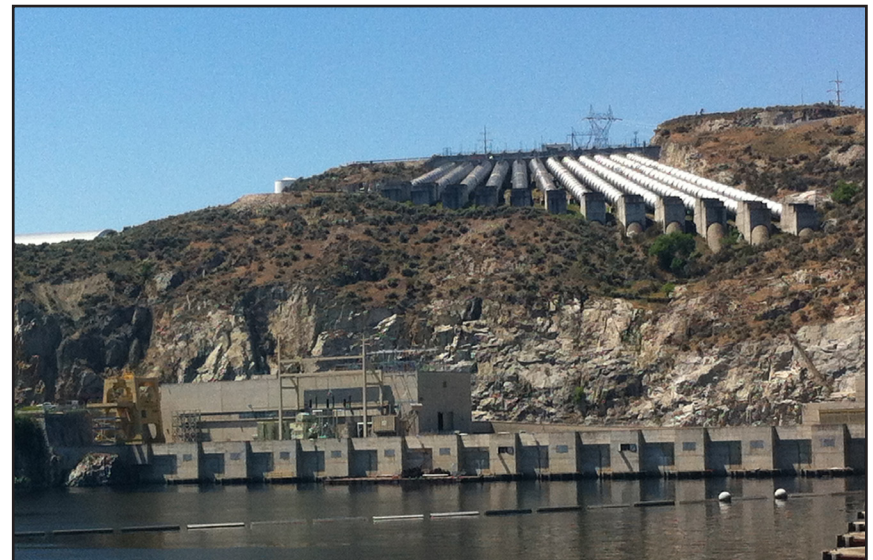
John W. Keys, III Pump-Generating Plant Named in honor of the former Reclamation Commissioner Completed in the early 1980s, the pump plant contains 12 pumps that lift water up the hillside to Banks Lake to serve as the source of water for the Columbia Basin Project. Six of the pumps are reversible and are also capable of generating power.
